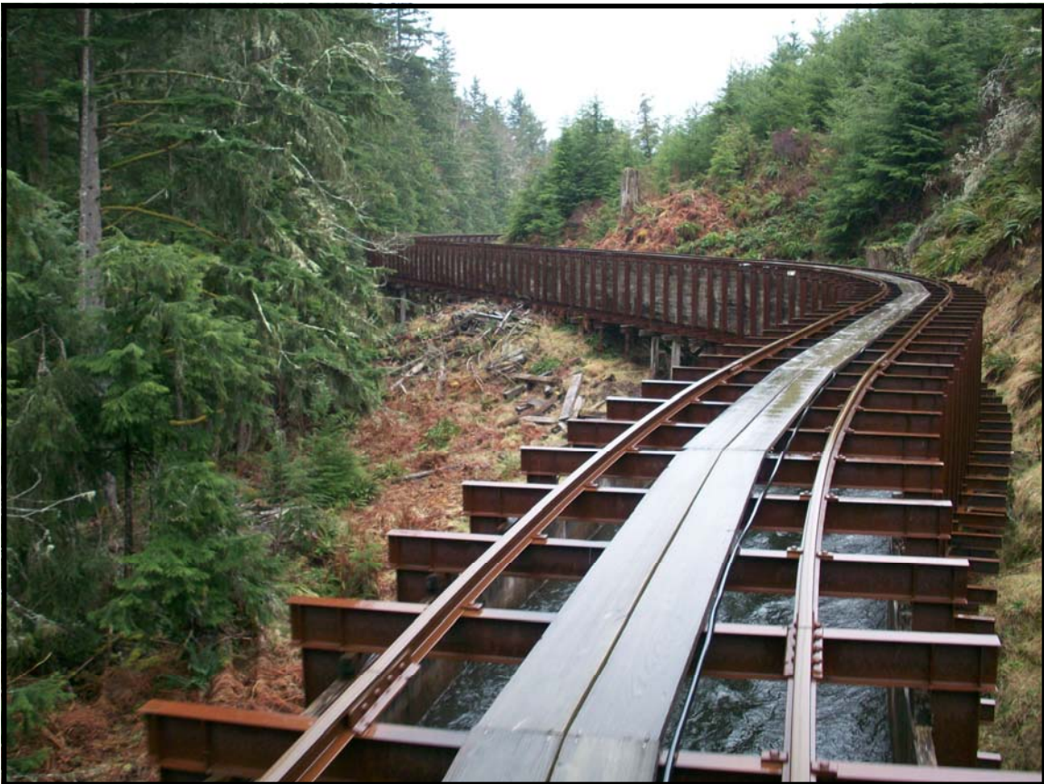
10.2 Mile Wooden Flume
