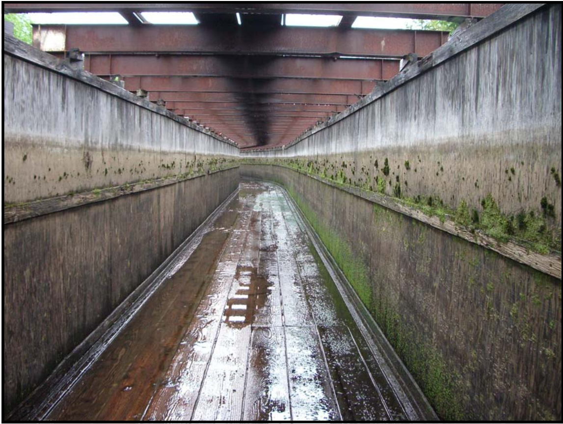
Existing Condition Inside Flume
