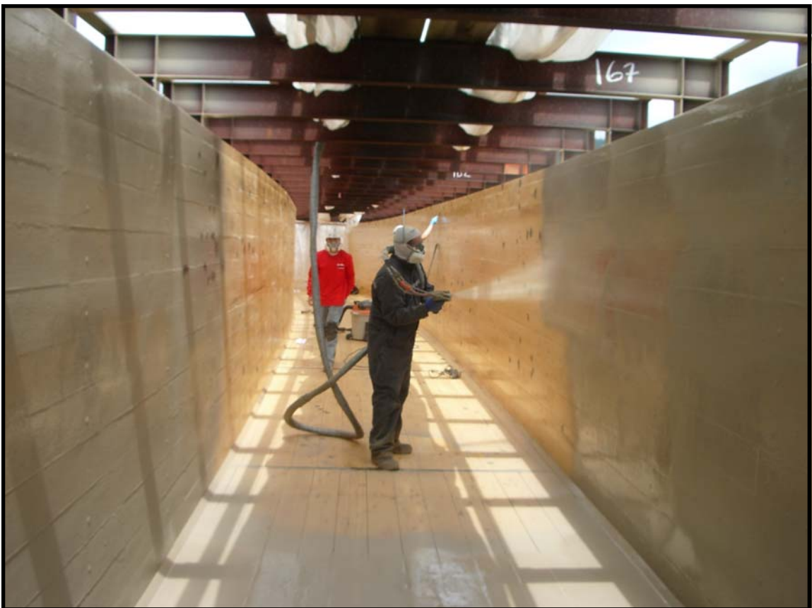
Spraying Polyurea Liner on Alaska Yellow Cedar
