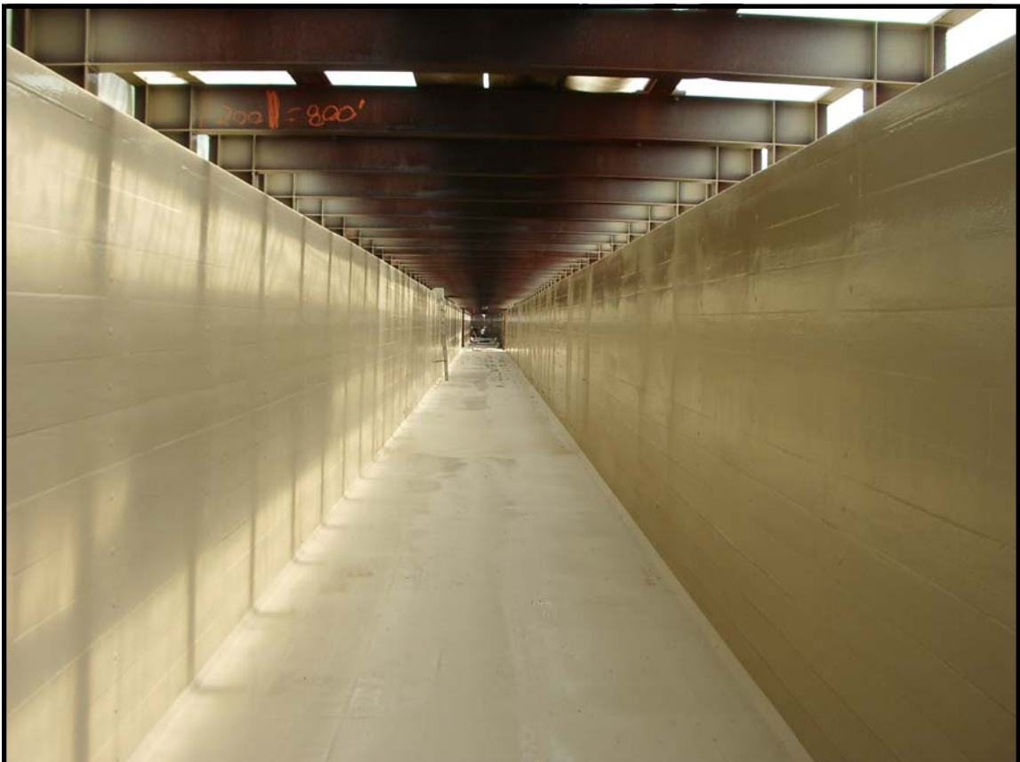
After Flume Repair: Alaska Yellow Cedar Lined With Polyurea
